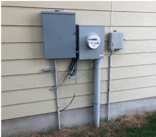
**Typical Underground Meter Loop**
